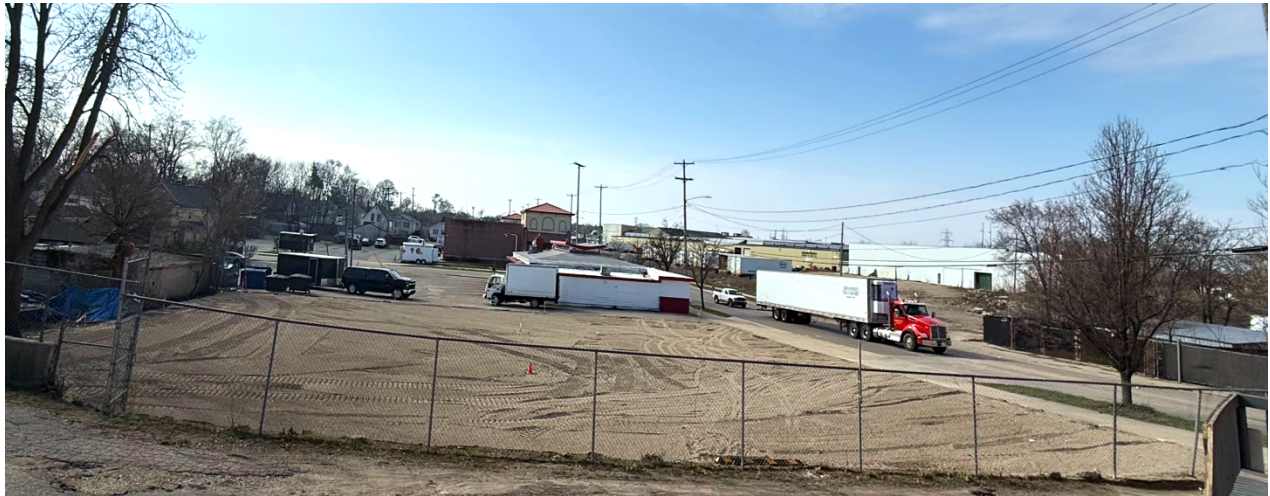
Ready for New Fence and Asphalt
