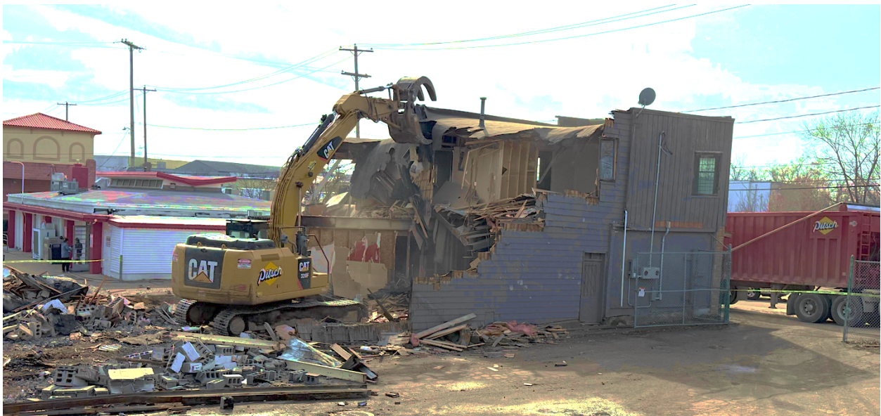
Demolition in Progress!
