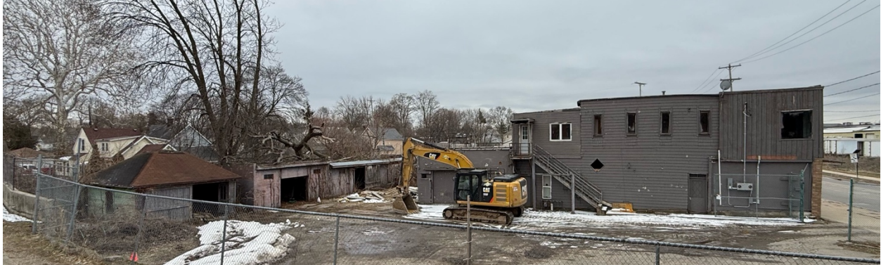
RPM New Property Prior to Demolition
